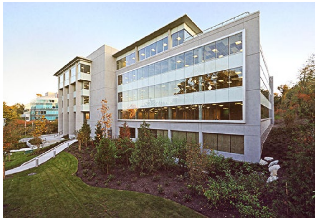
The LDB's new head office in Burnaby, BC is certified LEED Platinum. Pictured here nearing the end of construction in 2009.
